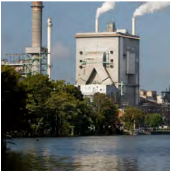
Domtar Corporation's Plymouth Mill in Plymouth, North Carolina
